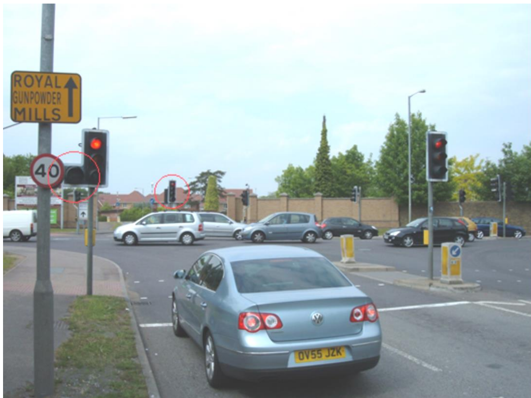
Figure 3: Meridian Way approach showing left turn filter green arrows (circled in red) before 2009 improvements
