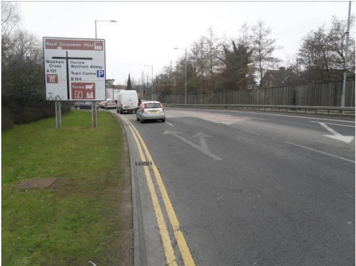
Photo 4 – Advanced directional sign on A121 Meridian Way northbound approach. Also shows worn directional arrow markings.
