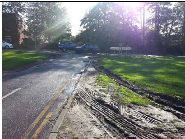
Photographs: Looking southeastbound on Lindsey Street link road
